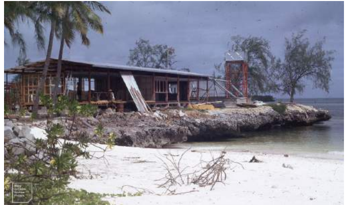
Research station under construction © Mary Gillham Archive Project
