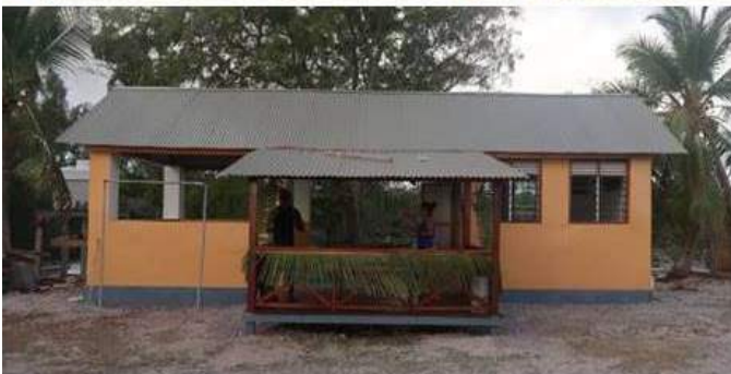
The old gym during and after renovations © SIF
