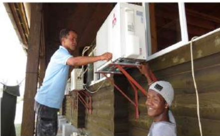
Installing the new energy efficient air conditioning units © C Quanz
