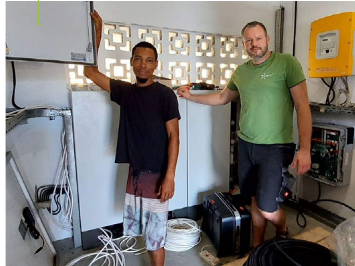
Trevor and Thomas replacing old inverters with new ones © Christina Quanz
