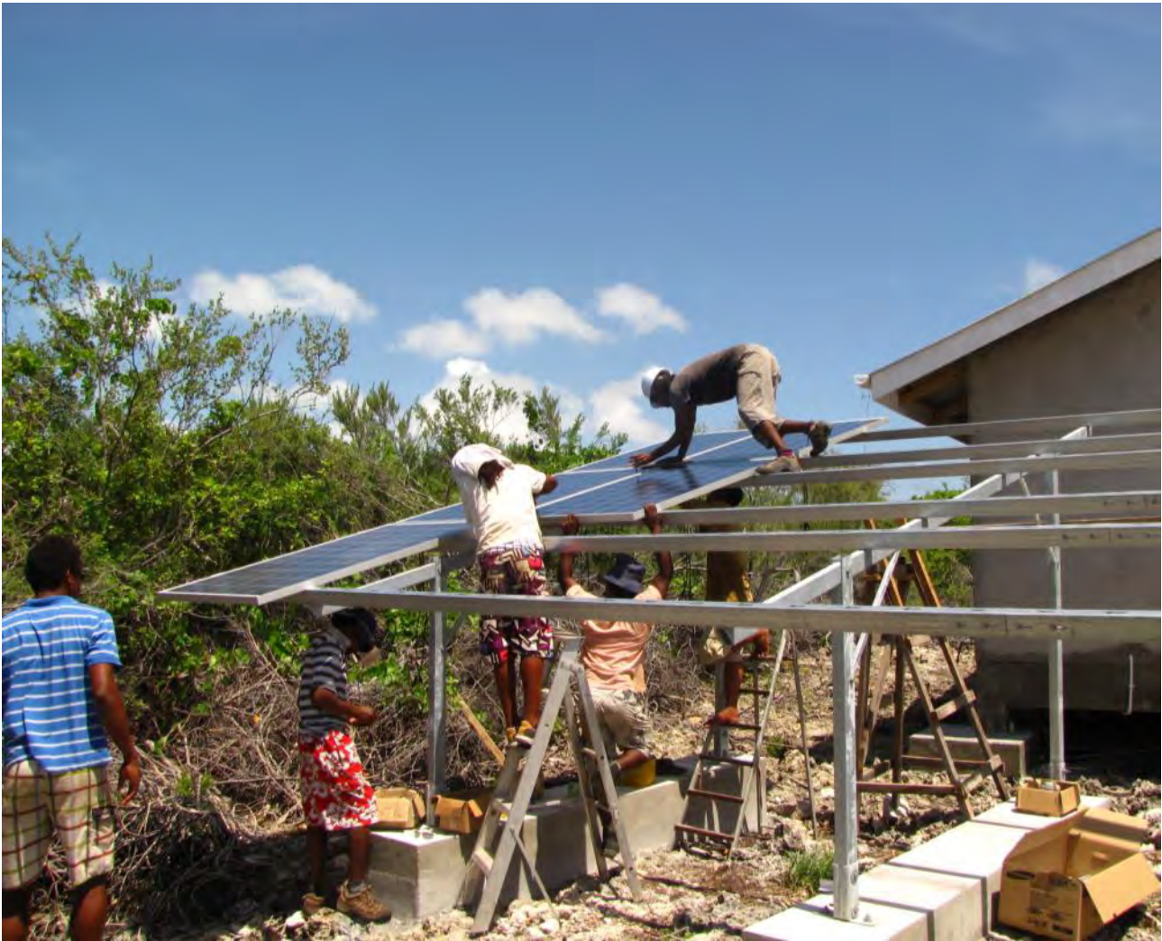
SIF staff on Aldabra assembling solar modules on mounting frame © Christina Quanz (March 2012)
